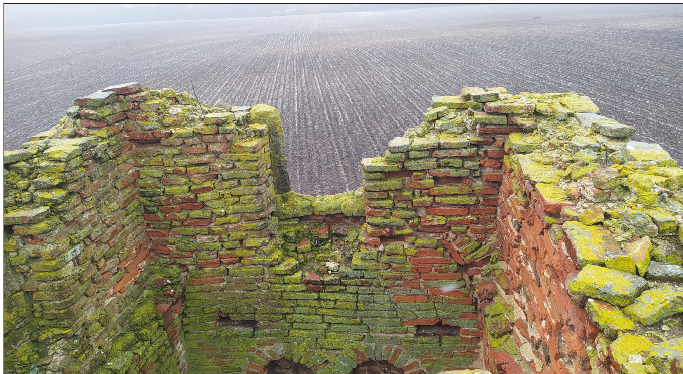
Fig. 12. Remains of the second-floor vault of the Romanesque tower
