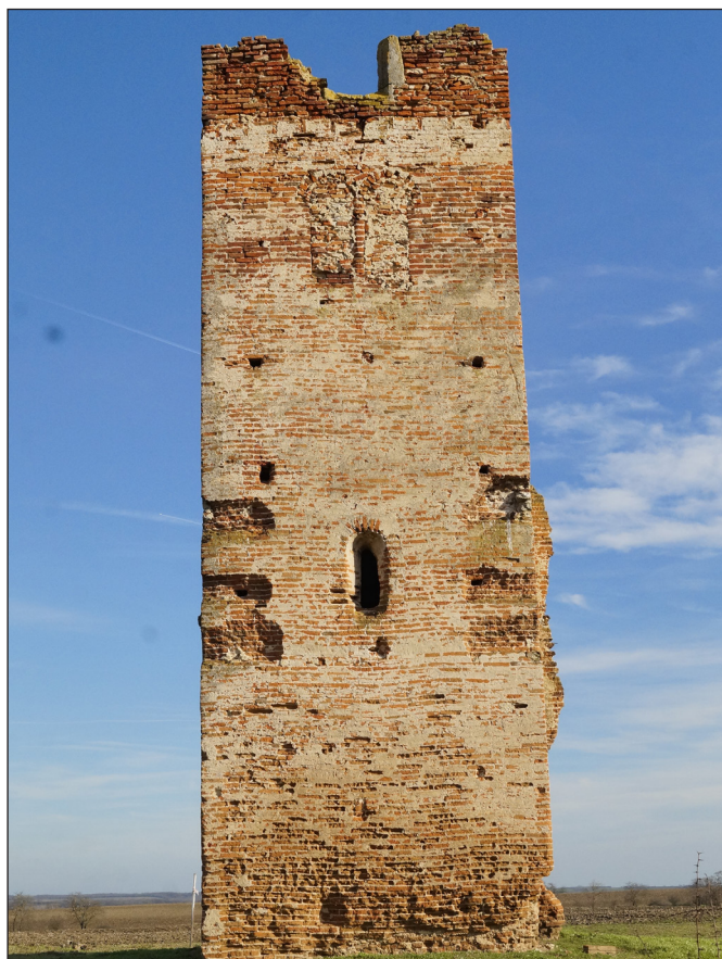
Fig. 1. South-western facade of the tower
