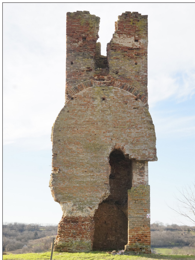
Fig. 4. North-eastern facade of the tower
