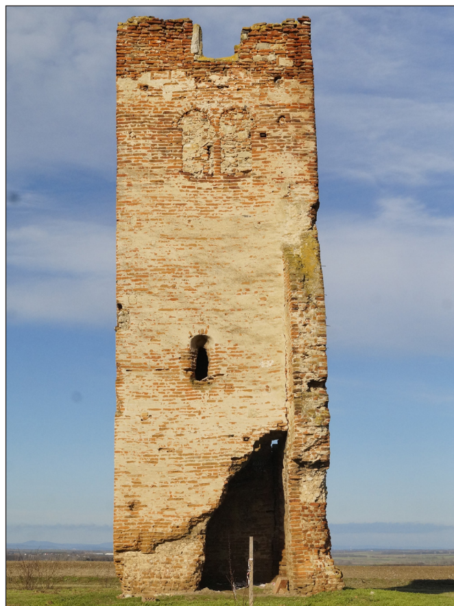
Fig. 2. South-eastern facade of the tower
