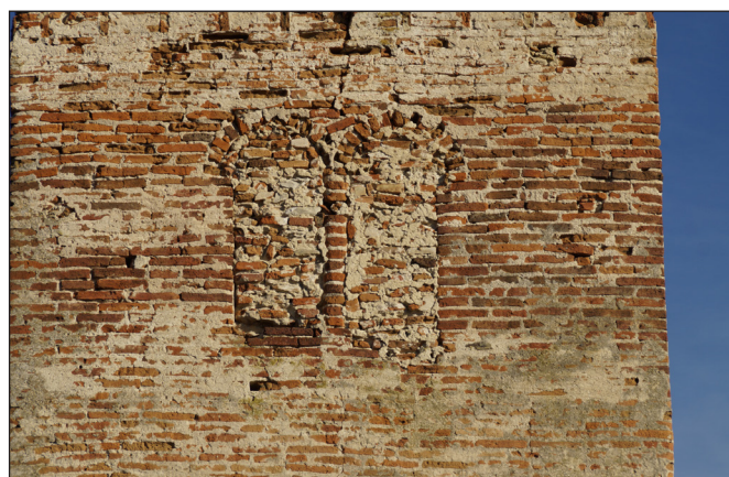
Fig. 7. External view of the second-floor window on the south-western facade
