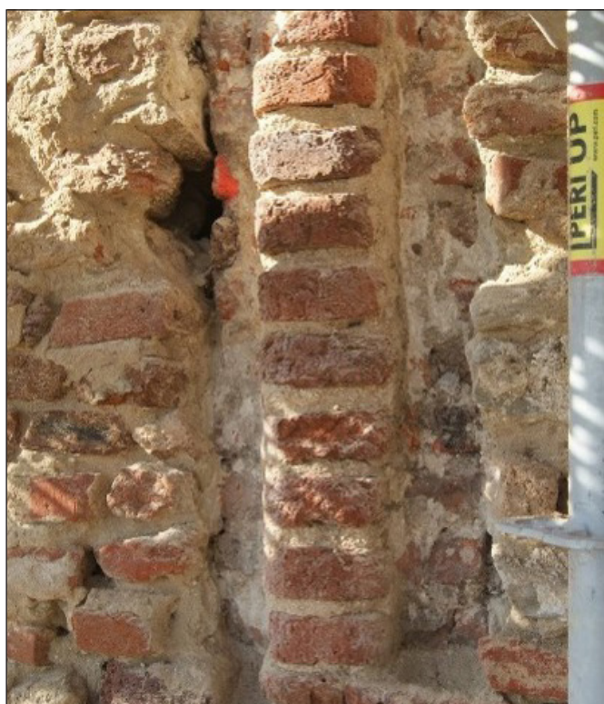
Fig. 8. Mullion after exploration
