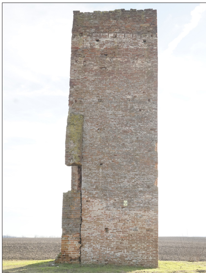
Fig. 3. North-western facade of the tower
