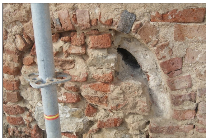
Fig. 9. Detail of the vault after research
