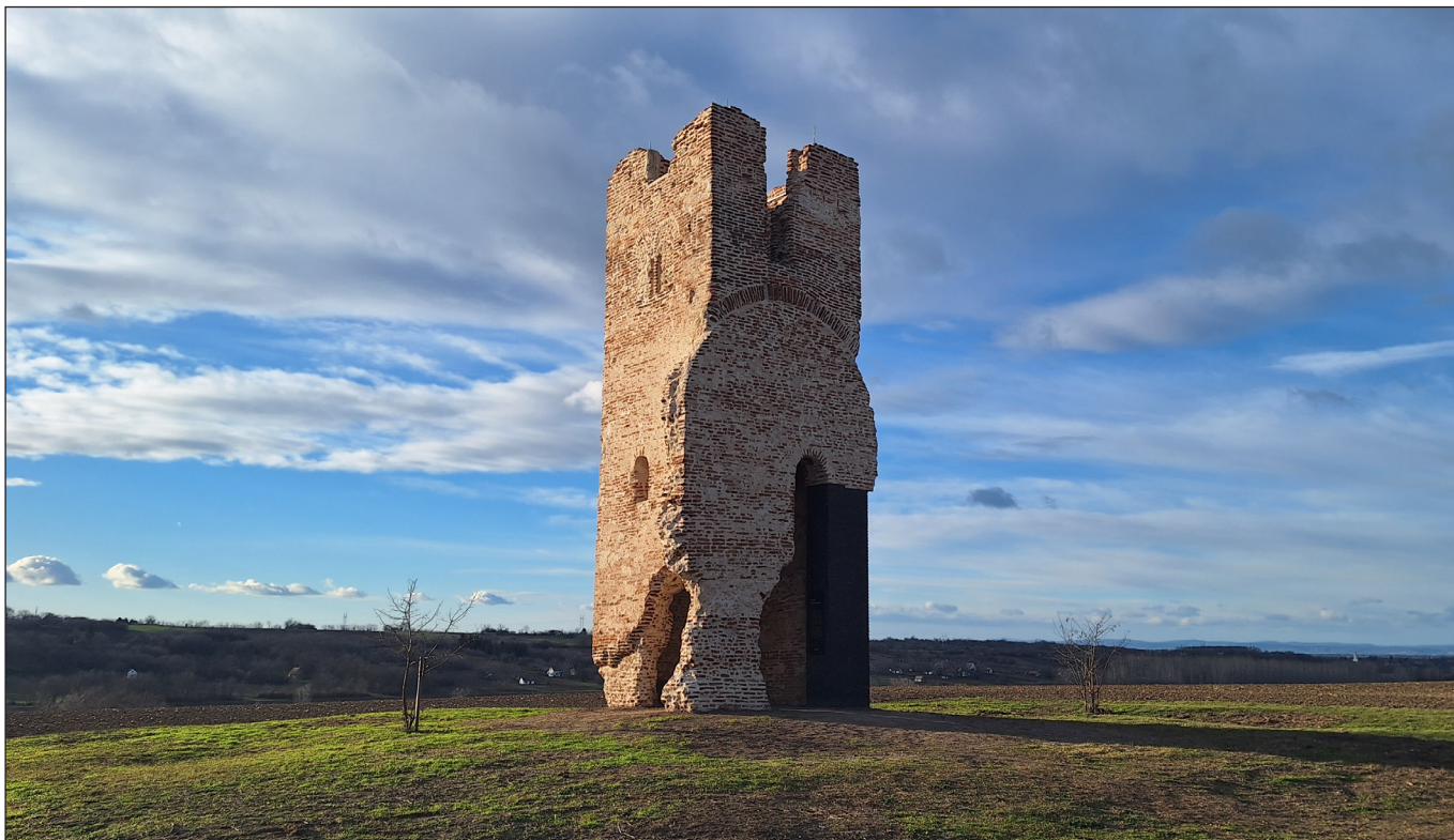
Fig. 15. The restored and conserved tower with the new corner pillar
