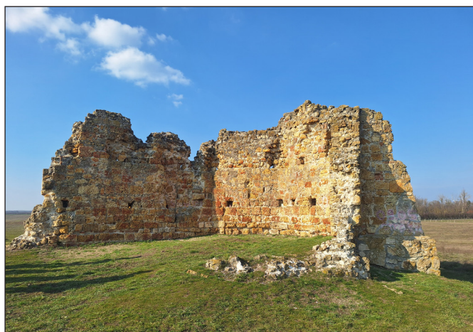
Fig. 8. The interior of the church before restoration – showing the heterogeneous infill masonry of the pillars from 1999 (photo: Bálint Kelemen)
