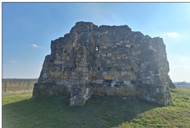
Fig. 7. The sanctuary viewed from the east before restoration (photo: Bálint Kelemen)
