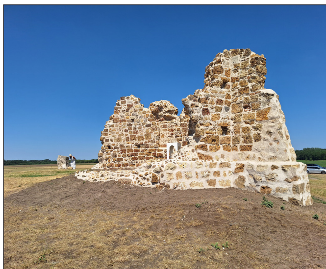
Fig. 10. The ruins after restoration – with a thin layer of plaster applied to the surface of the previous pillar reinforcements and new infill masonry (photo: Bálint Kelemen)
