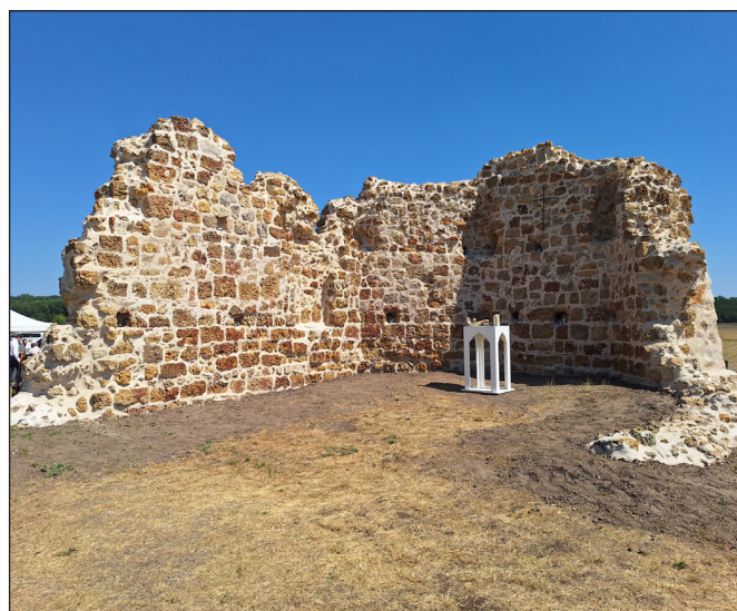
Fig. 11. The interior of the ruins after restoration – with the wrought-iron cross on the sanctuary wall (the temporary installation in place of the altar is not part of the restoration) (photo: Bálint Kelemen)
