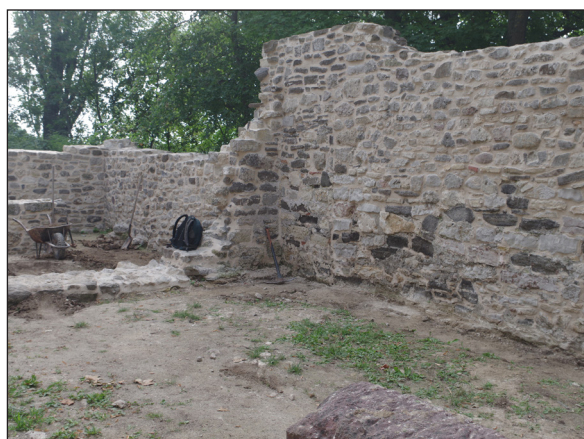
Fig. 17. The nave with the floor level deepened by builders but before excavation on 17 July 2023
