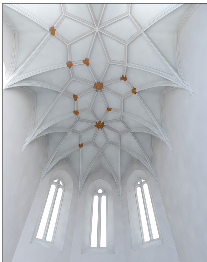
Fig. 24. Computer-aided theoretical reconstruction of the chapel of the Franciscan friary. The digitised carved stone elements of the vault are marked in red. SziMe3D AR project
