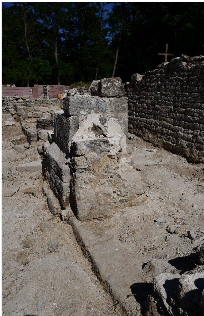
Fig. 25. The reinforced second pillar of the church's southern colonnade
