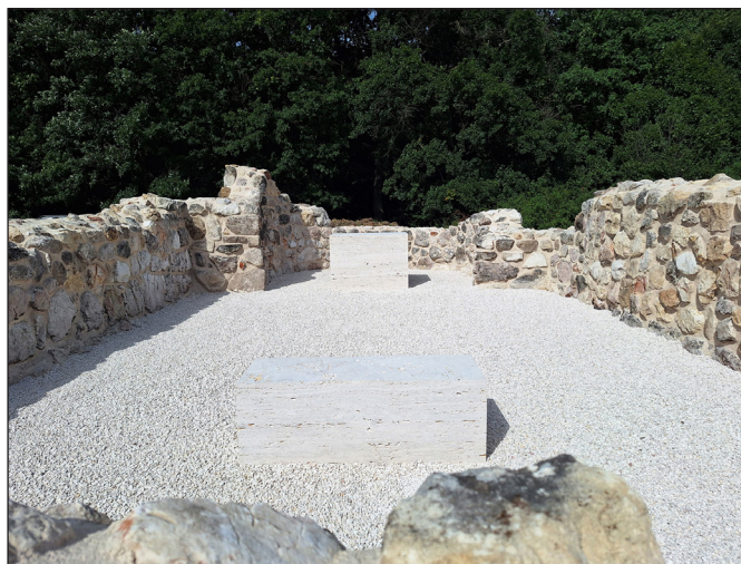
Fig. 5. The interior of the church with a limestone altar and a bench
