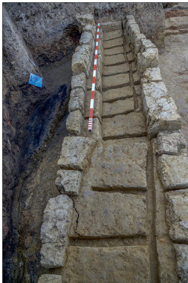
Fig. 10. Imprint of a completely decayed wooden beam in the core of the main dividing wall, made of unfired clay bricks Szolnok Castle, Trench 3, Ottoman palace (photo by K. Kozma, 2018; after KERTÉSZ 2021, 549, Fig. 574)
