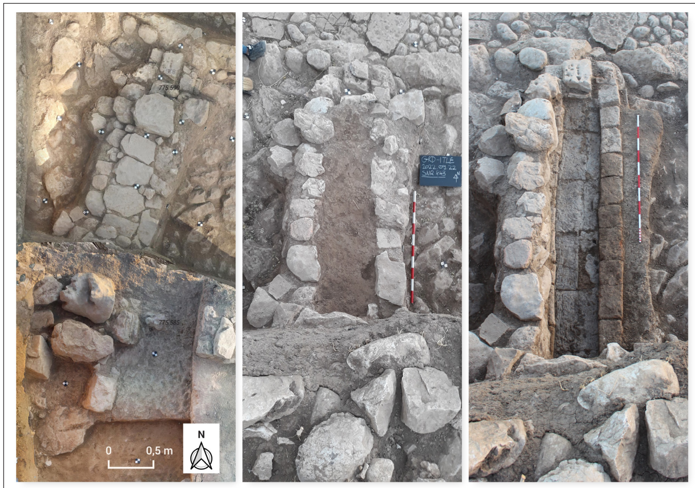
Fig. 11. Grd-i Tle, northern slope. The Hellenistic-Parthian drainage channel in subsequent stages of excavation in 2022. The bottom of the feature was made of fired bricks covered with bitumen, the top layers consisted of clay and stone rubble capped by large, flat blocks
