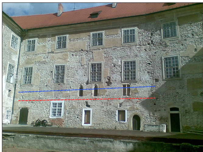
Fig. 3. Castle of Siklós, eastern wing, with a schematic indication of the raising of the inner floor level (survey by monument researcher Bartos György, 2009)
