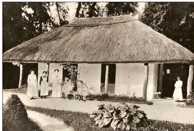
Fig. 5. 'Peasant house' in the garden of the Nádasdy castle in Nádasdladány, 1911 (source: Szalon Újság); its remains were found during the test excavation by Dóra Hegyi and Zsófia Nádaï (HEGYI, KLAGYIVIK & NÁDAI 2017)
