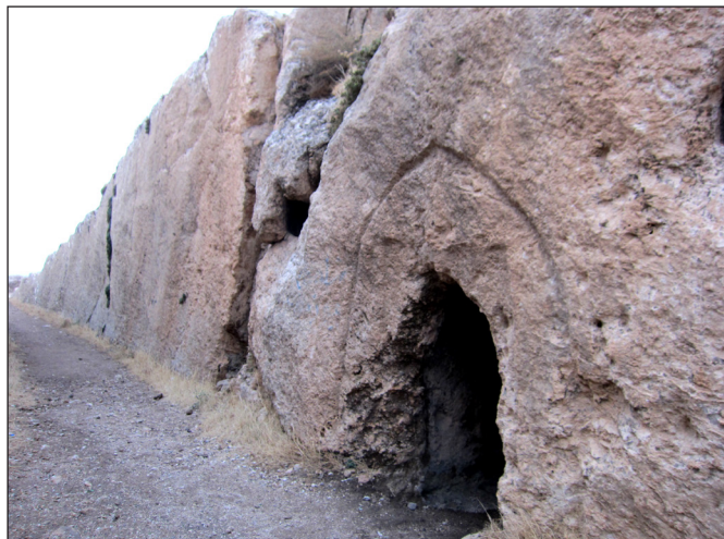
Fig. 10. Entrance of a room carved into the rock in Akre Castle
