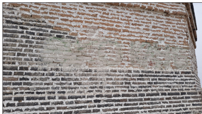
Fig. 15. Structure of the wall of the restored stupa
