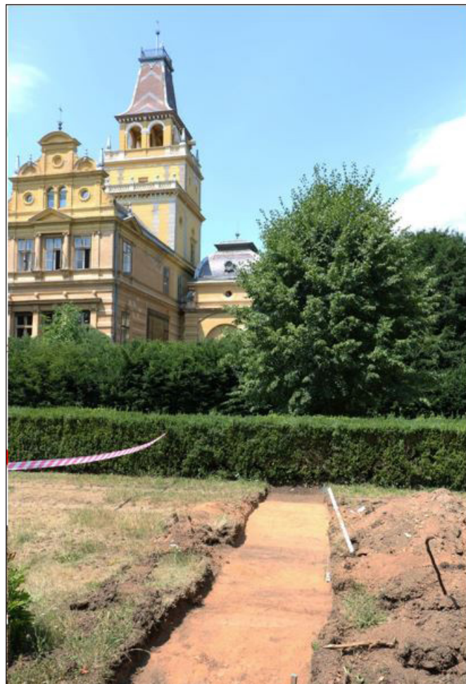
Fig. 17. Foundation of the pathway in front of the castle's southern façade
