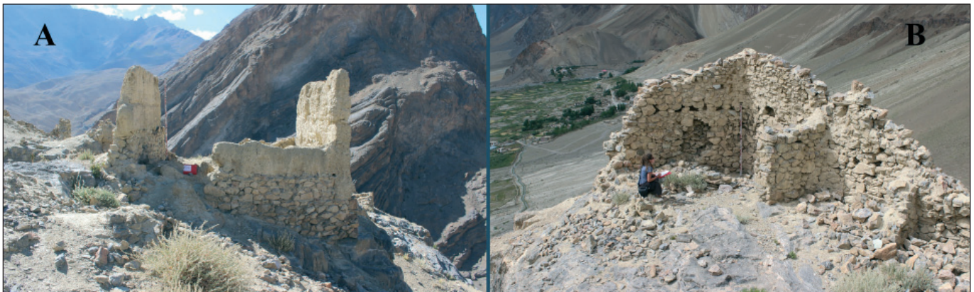
Figure 11: The northern (B) and the western (A) bastions
