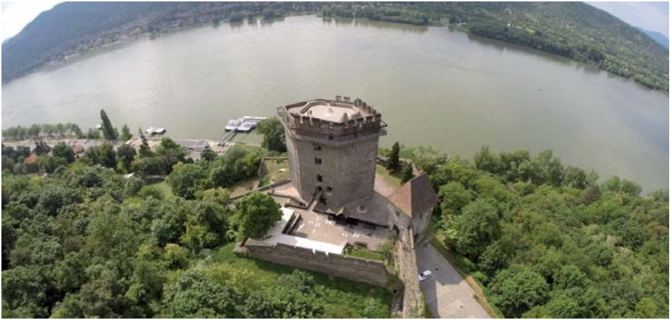
Figure 1. The 32 m high Solomon Tower with the external ramp at the top
