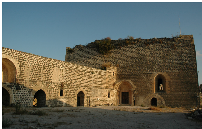
Fig. 2: The Hospitaller chapel as seen from the central courtyard of the citadel, with its northern doorway in the centre and vaulted ranges I.1.D on the left (photograph: Balázs Major)
