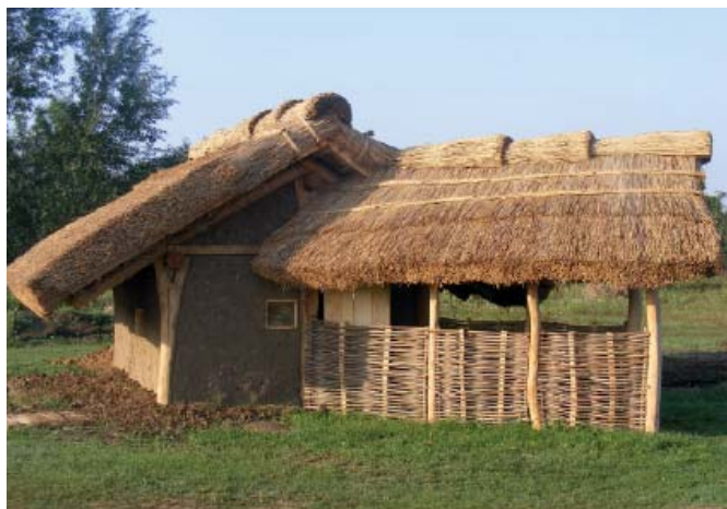
Fig. 5: Reconstruction of a house with a projecting roof supported on vertical walls from Szamoskér
