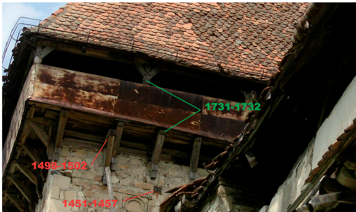
Fig. 8: Dated elements from the western bell tower in Drăușeni
