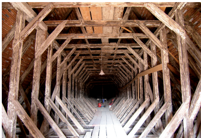
Fig. 4: View of the roof structure in Sibiu
