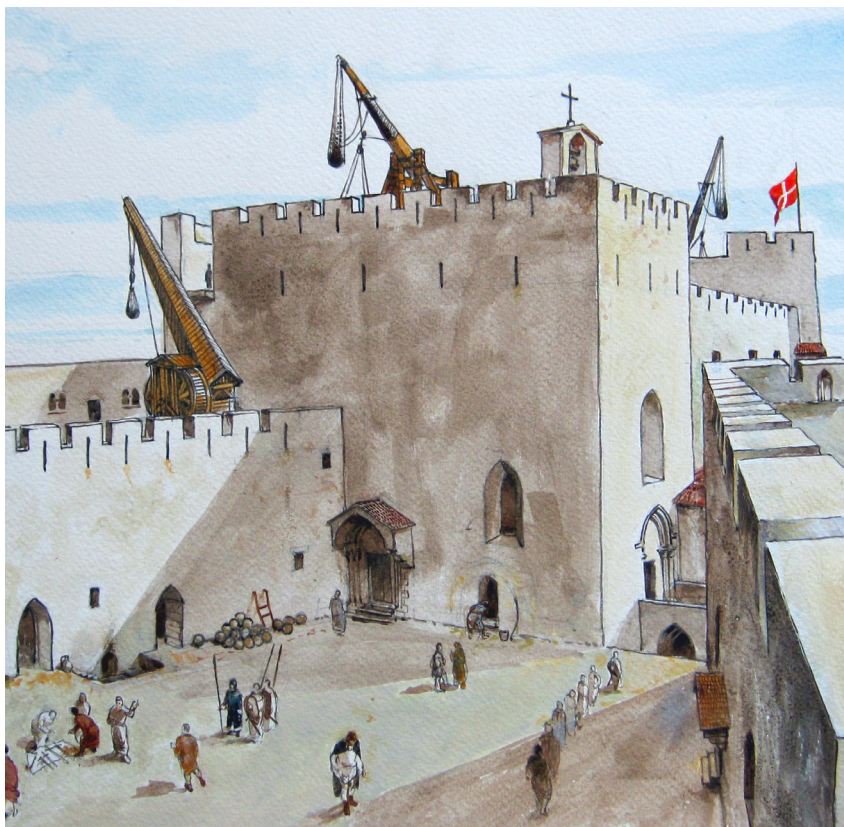
Fig. 3: Reconstruction of the courtyard corner adjacent to the chapel with the crane
