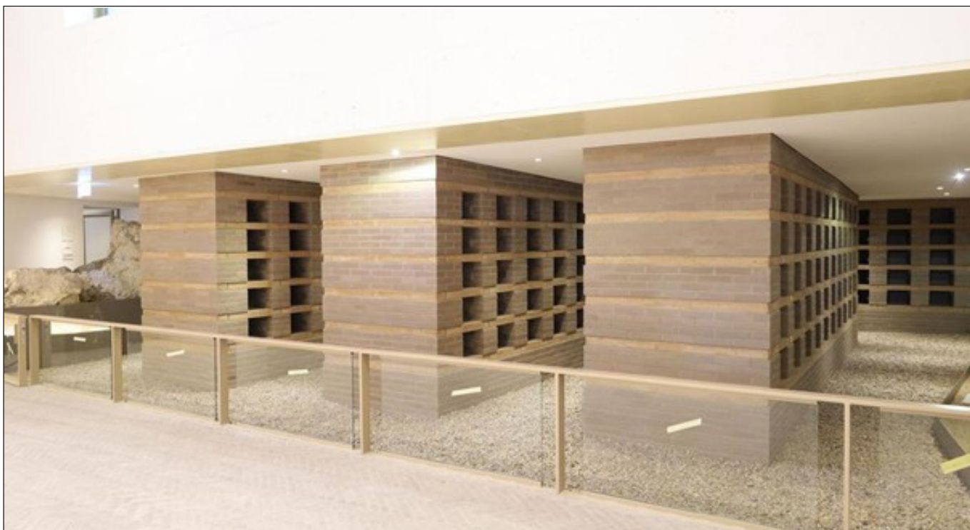
Fig. 5. Ossuary in the basement of PETRI. Berlin's medieval "natives" will be reburied here. Mud bricks will be used for walling up the holes. © BM / Christof Hannemann
