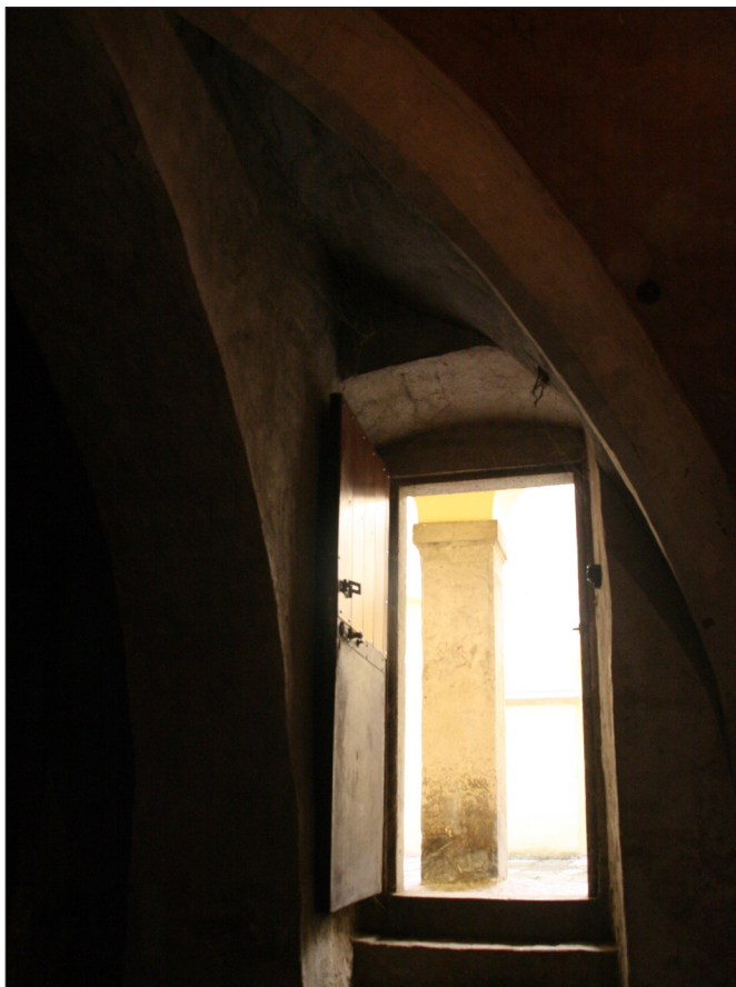
Fig. 5. Remains of the ground floor vaulting in the tower under 7 Kolostor Street in Sopron. (photo by Gergely Szoboszlai)
