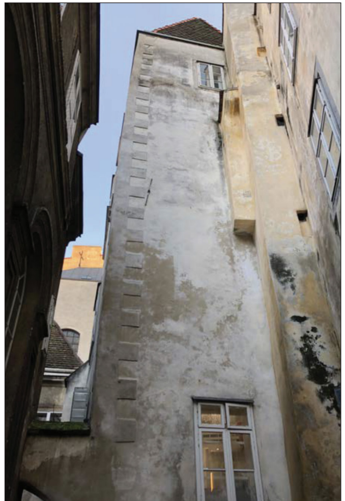
Fig. 10. The tower of Griechengasse 14 in Wien the symbolic plaster masonry (photo by Gergely Szoboszlai)
