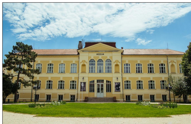
Fig. 2. The Savaria Museum after renovation in 2019
